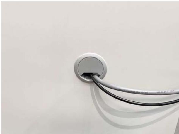
**Fig 1. Power lead and water feed line passed through the lowest 54mm port hole**
