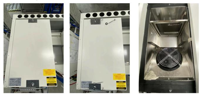
Undo the top cover of the conditioning duct of the cabinet using 10mm spanner or socket .
