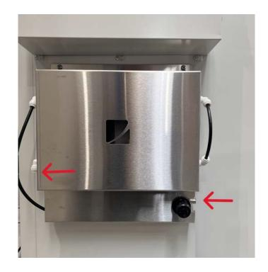
With the pressure released in the hose, disconnect the water inlet to the pressure reduction valve and the water outlet to the cabinet on the filter pack.
