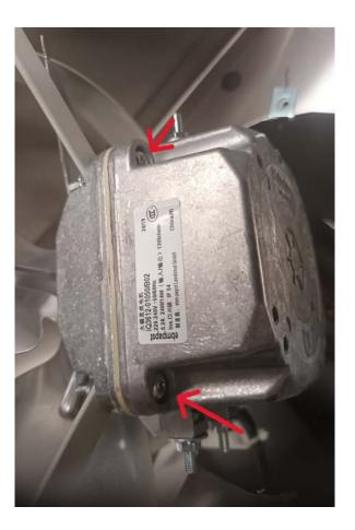
Once the fan motor is connected to the original wires, reattach it to the bracket using the four bolts in the corner of the motor. Then replace the motor into the shroud by installing the four fixing screws as shown below.
