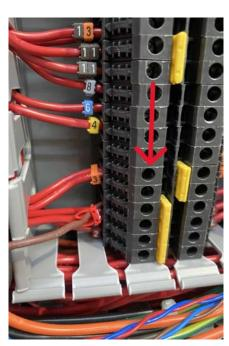
Unscrew the fixing screw and then place the red wire into the sample fitting on the terminal block where either the brown and blue wire is currently fitted and remove the wire.
