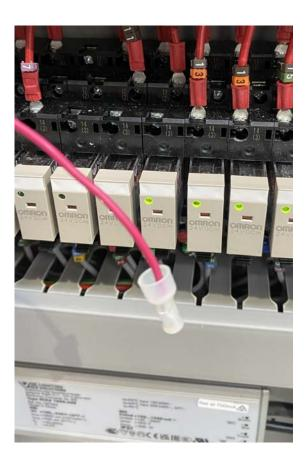
Taking both the low speed and high speed wires fit them both into the terminal block together. Re tighten the fixing screw to secure the wires in place.
