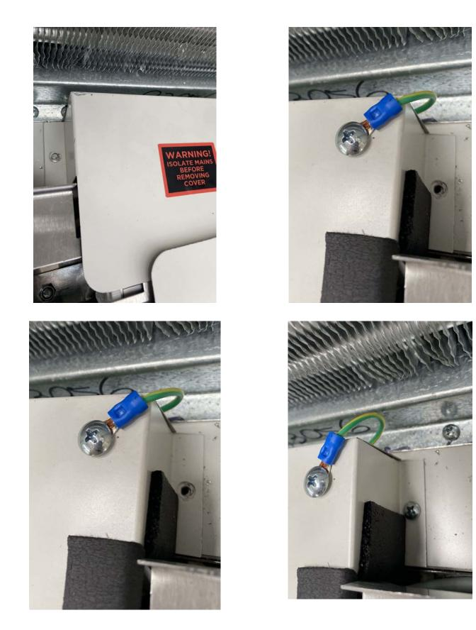
Place the cover back over the controller and line up the holes. Once they are lined up, fix the cover in place with the screws removed earlier.
