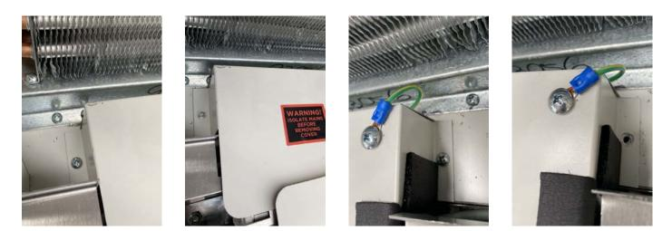
To remove this plate, undo the screws on either side of the plate. You DO NOT need to unscrew the green earth wire on the back of the plate.
