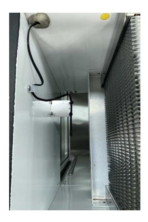
Attach the black wire under the white wall bracket and fasten the sensor to the metal bracket with cable ties.
