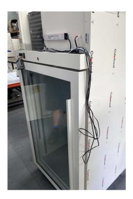
In order for you to have complete access to the sensor wires, you will need to remove them from under the fascia and move them to the side. This will provide you with sufficient slack to adjust the wires as required.
