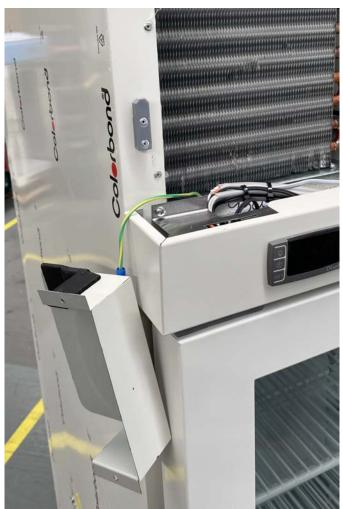
After removing the screws, lift the plate to reveal the controller. The plate can be placed behind the controller on the evaporator coil or to the side.
