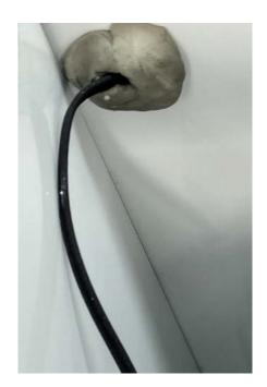
Insert the new Dixell sensor into the evaporator enclosure. Seal the surrounding holes with the original putty.
