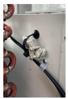
To remove the Dixell sensor, first cut the cable ties that fix it to the bracket. Then, carefully remove the putty around the conduit that the sensor wire passes through from the evaporator enclosure to the front of the fridge. However, make sure to keep the putty as you will need it later to seal the area around the new sensor.
