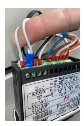
The bottle sensor, door switch and the return air sensor (Black NTC Dixell sensor) are connected in the same common terminal 11 via pin crimp connector. To remove this you have to cut the connector. Once you cut this wire, thread it through the conduits leading into the evaporator enclosure and then this will allow you to remove the bottle sensor completely. You will also have to remove the other wire from terminal 10.
