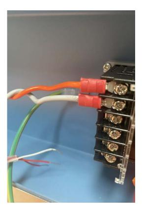
To connect the new sensor to the controller, strip about 1-1.5cm of the plastic sheath from the end of the PT100 wires, as shown.
