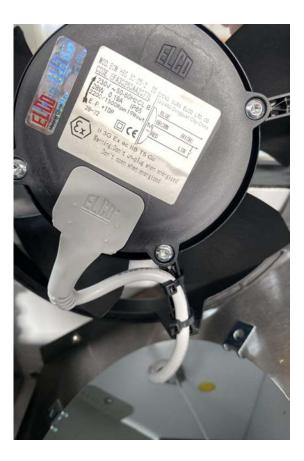
Connect the power cable to the new fan and secure it with the supplied cable ties.
