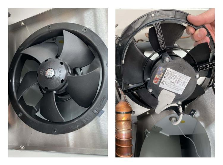
Remove the screws holding the evaporator fan in place (there are four in total). This will allow you to pull out the evaporator fan.
