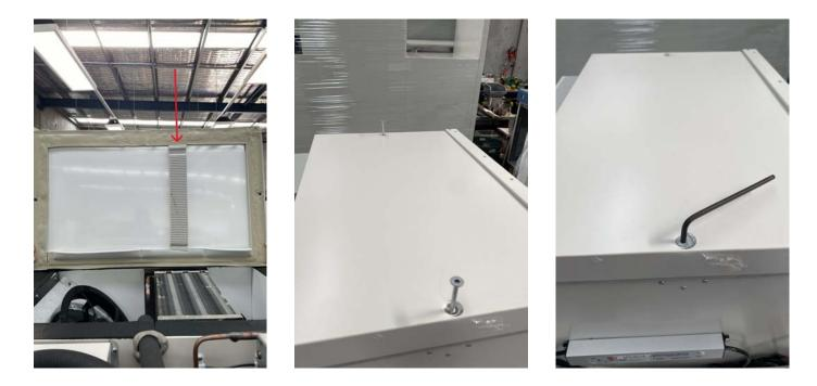
To install the evaporator enclosure lid, ensure that the strip of foam running across the top is placed over the evaporator coil. This helps to cool hot air through the evaporator, rather than letting it pass above it. Once the lid is in place, screw it down securely.
