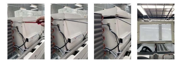
To open the evaporator enclosure, take a large flat head screwdriver and insert it between the foam tape and the top of the enclosure. Then, gently lever the screwdriver upwards to break the seal. This will allow you to remove the lid from the evaporator enclosure.
