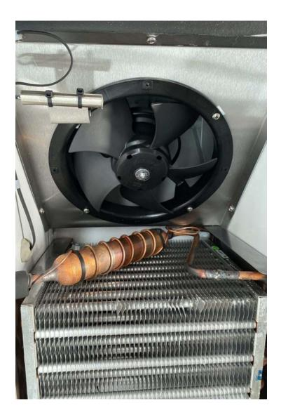
When you remove the cover, you will see the evaporator coil, the evaporator fan and the silver tube that contains the Dixell hot key sensor.
