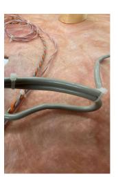
Once the D-Series motor has been connected, re-insert the wires from the new D-Series Motor into the plastic connector and pull the tabs down. Using cable ties, refix the wires together.
