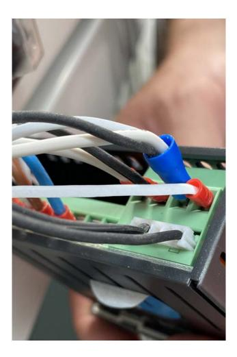
Insert the white plug of the new sensor into the back the Dixell Controller
