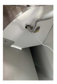
Remove the putty around the conduit that the Dixell sensor wire goes through but do not discard it (you will need this later to seal the area around the new sensor).
