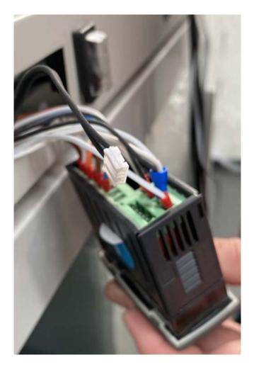
The Dixell Hot Key sensor is connected to the Dixell controller via a white connector. To disconnect it, gently pull the connector out.
