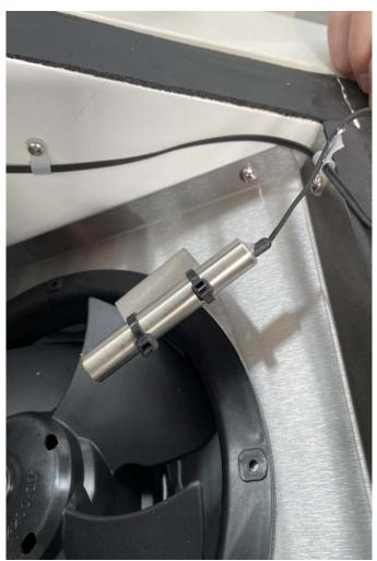
Gently push the sensor tip back into the silver tube until it is inserted about 1 to 2 cm.
