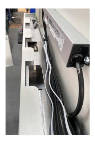
Once the controller is in place, you can then place the wires under the fascia neatly.
