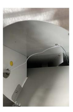
Once the screws of the evaporator fan are removed (there are four in total), you can pull out the evaporator fan. Through the cut out where the evaporator is housed you will see the white wire of the bottle sensor.
