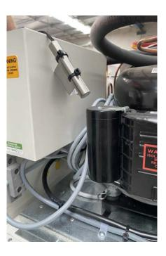
Undo the Dixell hot key sensor housing using a small Philips head screw driver and place it to the side.
