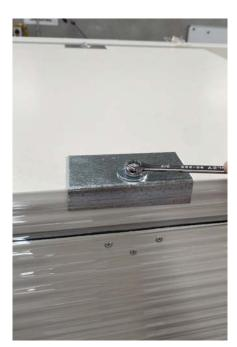
Using a 5mm Allen Key, remove the screws that secure the cover of the evaporator enclosure.
