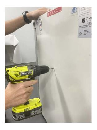
Use the 5mm drill bit to create a pilot hole from the outside.
