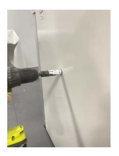
Using the 20mm hole saw, drill through the pilot hole from the outside.
