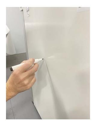
Mark the location of the pilot hole with a suitable marker. Please ensure that port hole will be away from the Shelvex strips, other internal fixtures and walls.
